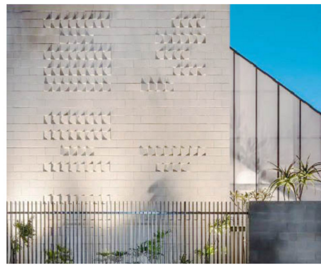
BLK - 01 FEATURE WALL WHITE POLISHED MASONRY BLOCKWORK - ROTATION
